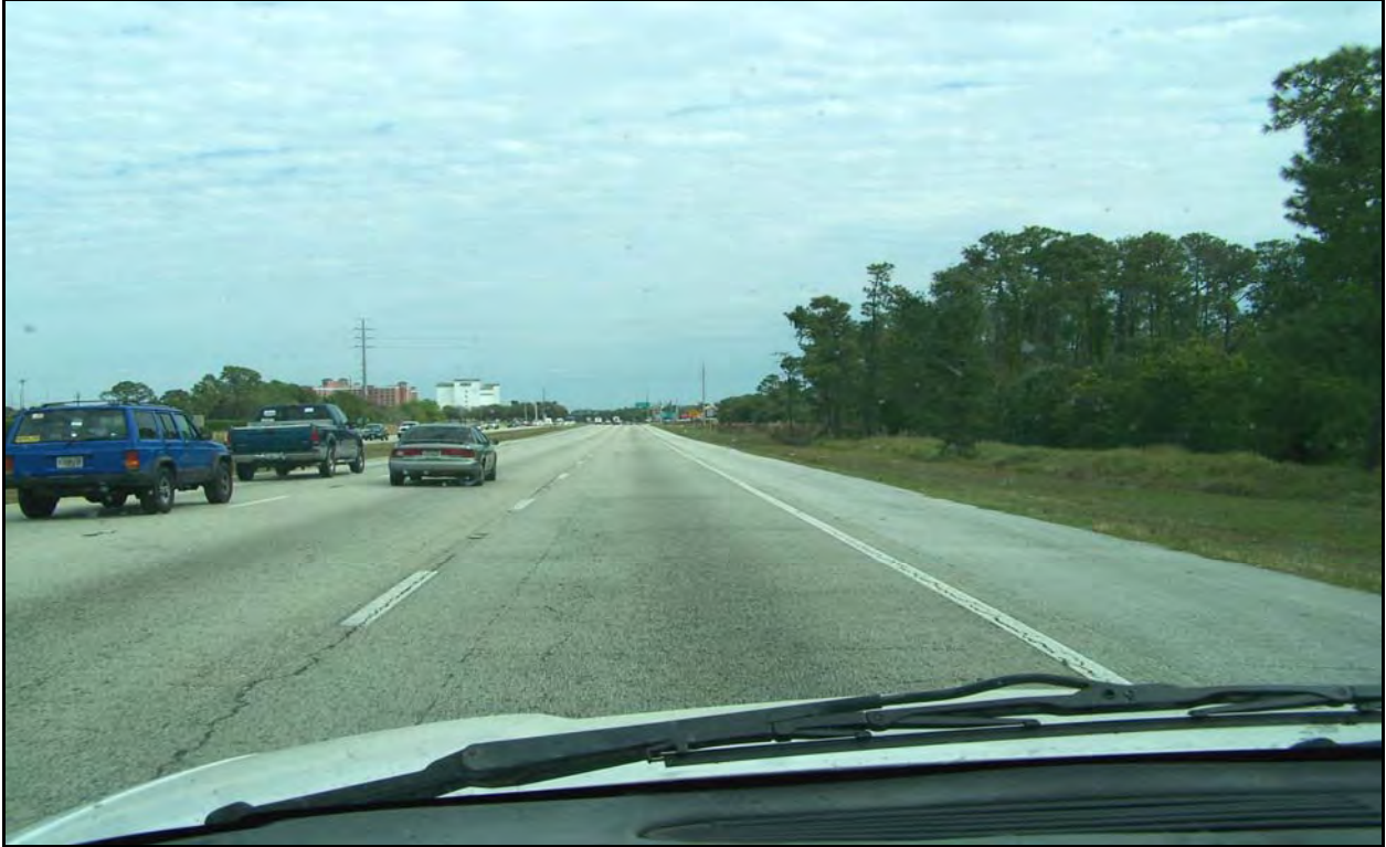
Photo 5: SR 536 eastbound near MP 1.700. Both the R2 and R3 lanes have moderate to severe cracking distress from MP 1.018 to the end of the project at MP 2.034.
