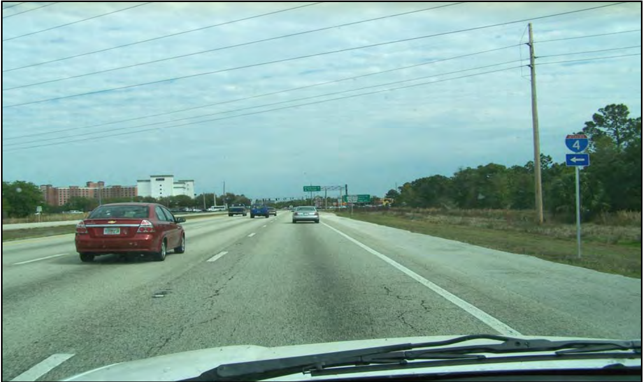
Photo 6: SR 536 eastbound near MP 1.900. This photo shows more of the cracking in the R3 lane.
