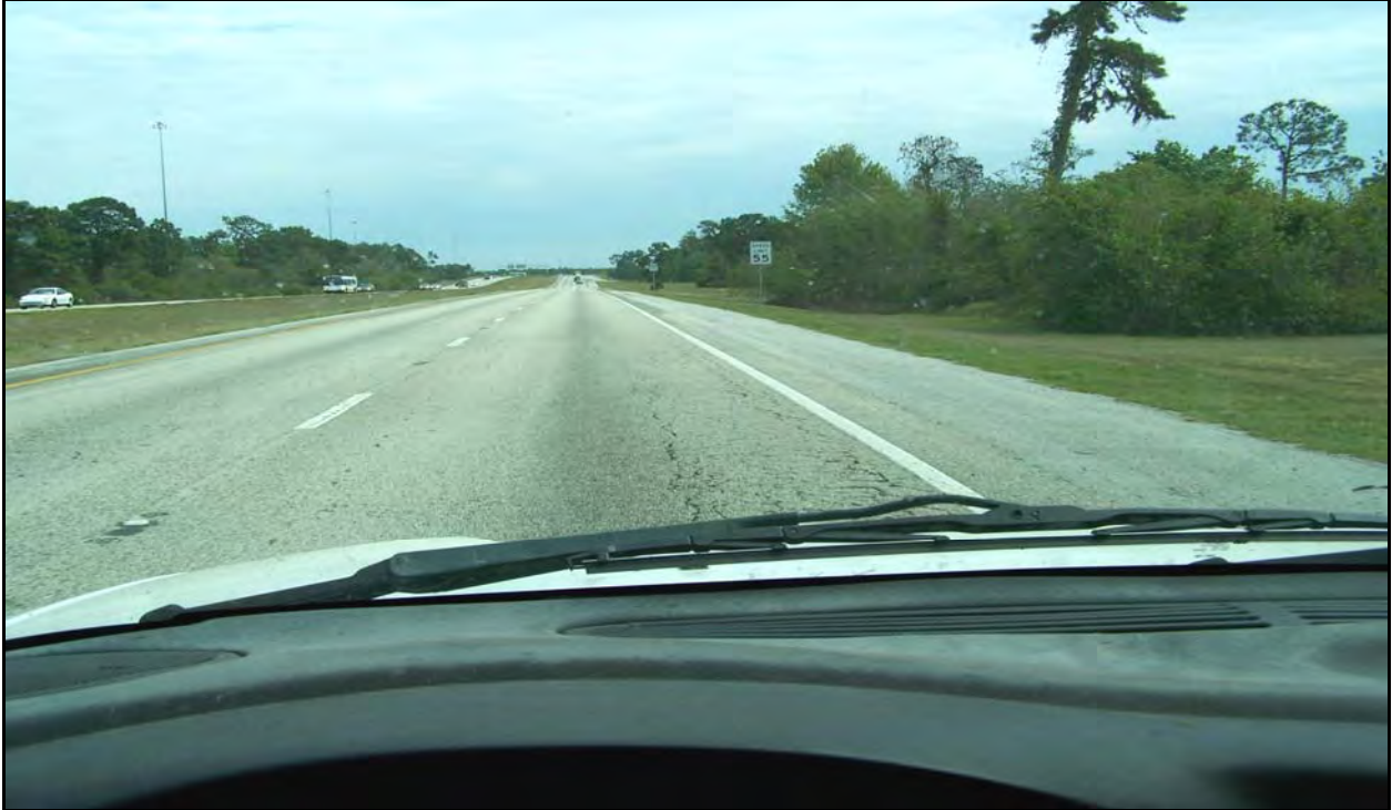
Photo 1: SR 536 eastbound near MP 0.130. This is an example of the severe pavement deterioration in the L2 and R2 travel lanes within the project limits. These lanes are heavily used by tour and transit buses going to and from the Walt Disney World theme parks.
