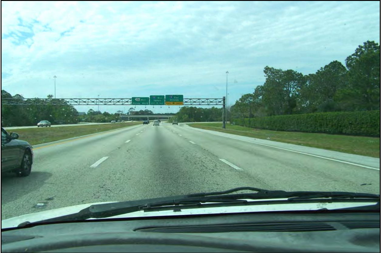
Photo 9: SR 536 westbound near MP 1.184. This is an example of the moderate to severe alligator cracking distresses in the L2 lane within the project limits.
