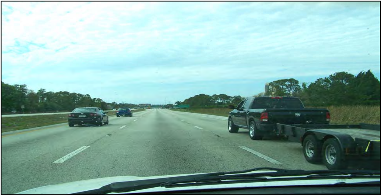
Photo 10: SR 536 westbound near MP 1.869. Typical condition of the westbound roadway.
