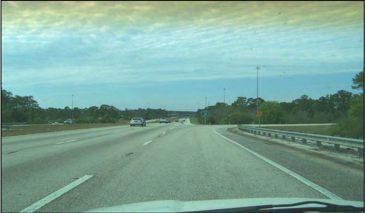
Photo 7: SR 536 westbound near MP 0.539. This is the last exit on the westbound roadway before entering Walt Disney World. There are no median crossovers after this milepost.
