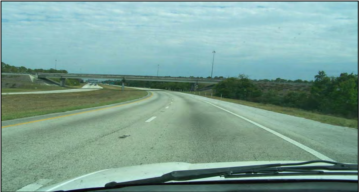
Photo 2: SR 536 eastbound near MP 0.740. The outside paved shoulders within the project limits are wider than the 4 foot shoulders seen on roads similar to this one. The inside paved shoulders have an FC-5 surface course. The outside paved shoulders have locations that have an FC-5 surface course, and some that do not have a friction course except for an overlap from the outside travel lanes.
