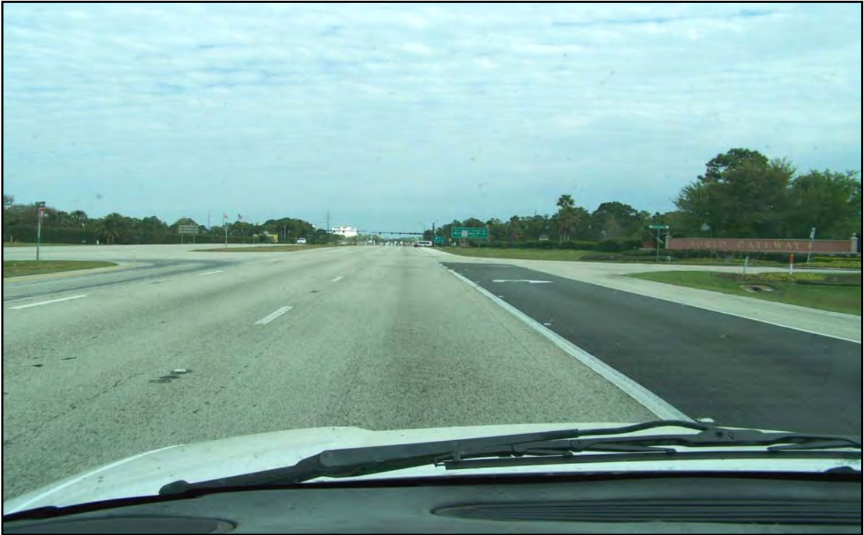
Photo 3: SR 536 eastbound near MP 1.305. This is in the R3 outside travel lane. Note the pop-outs of aggregates from the FC-5 friction course in the wheelpaths. The new asphalt in the right turn lane is a patch.
