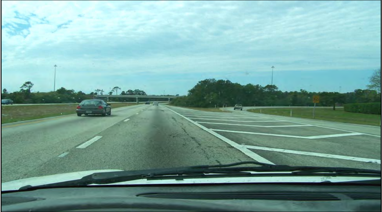
Photo 8: SR 536 westbound near MP 1.064. This is an example of the raveling distresses seen in the L2 lane.
