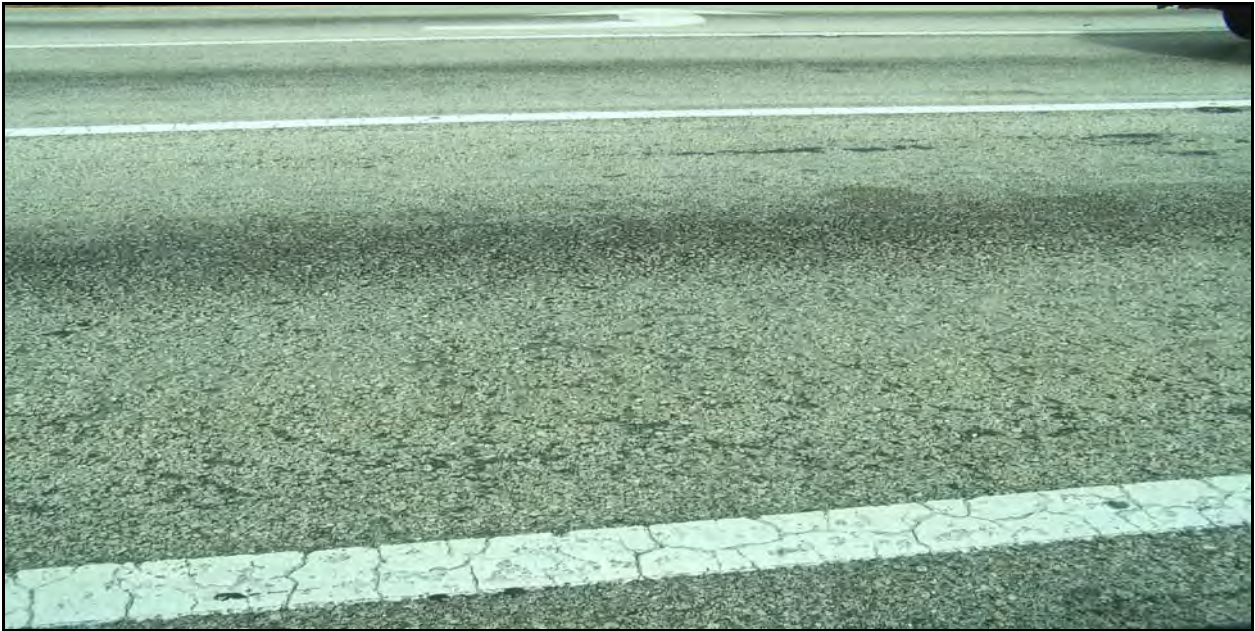
Photo 4: SR 536 eastbound near MP 1.515. This is a close-up of the pavement distress in the R2 lane. Note the cracking and severe raveling in this lane.
